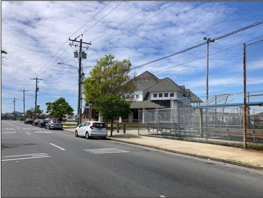
Northwesterly View of Subject Site
