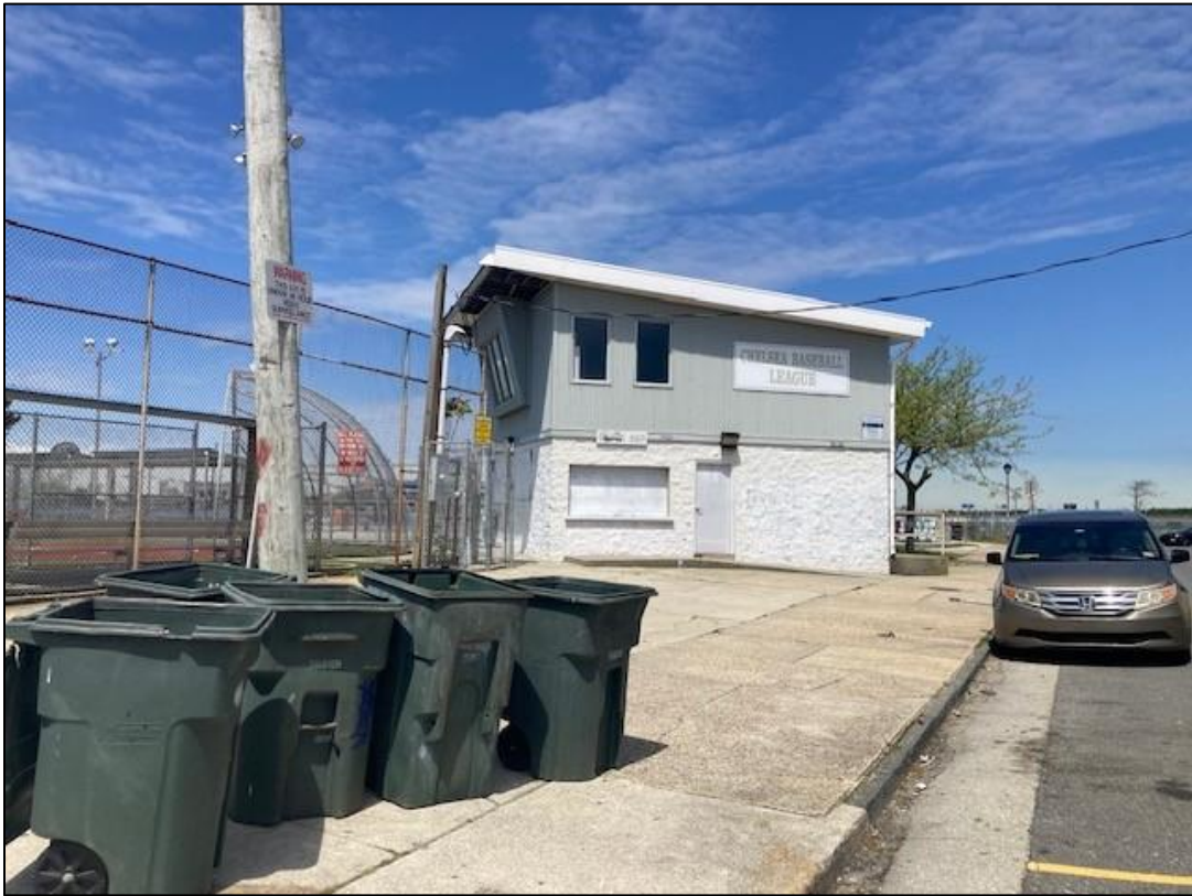
Northerly View of Subject Building (Building Not in Easement Area, Land in Foreground in Temporary Easement Area)
