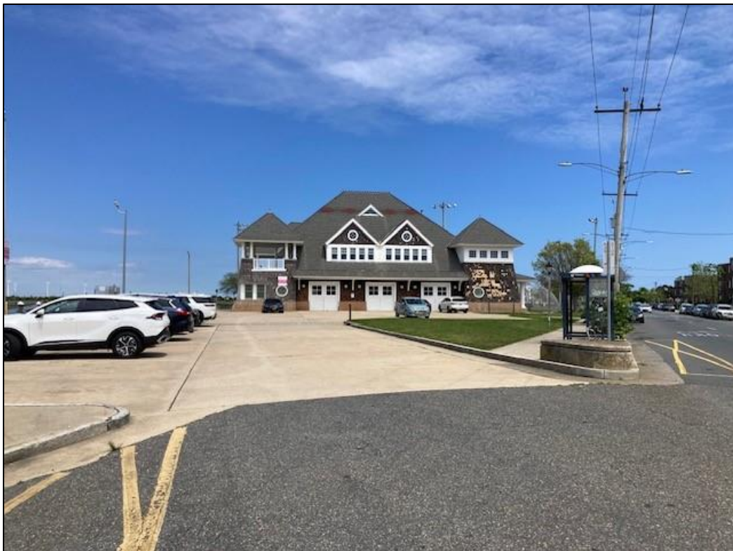
Northeasterly View of Subject Site
