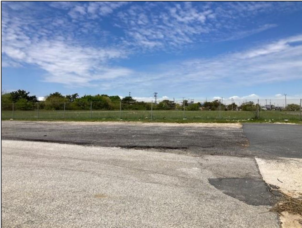
Westerly View of Permanent Easement Area Toward Temporary Easement Area from Boat Ramp Area
